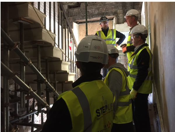
Scaffolding supporting the cantilevered stairs for repair
