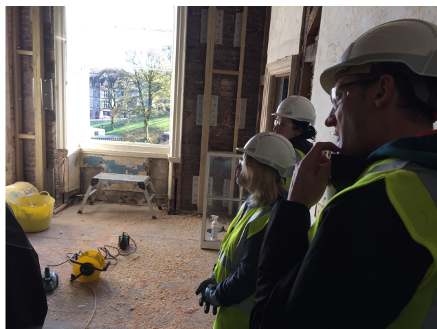
Sash window restoration
